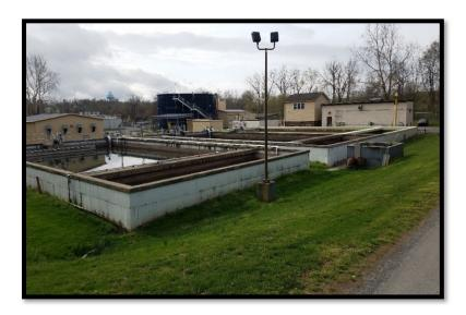
aerobic digester tank was added to the facility during an upgrade in 2005. The digester tank was built to provide additional sludge processing time and increased storage capacity in an effort to produce higher quality solids. Additionally, denitrification filters were installed at the facility in 2016, which included chemical addition facilities for coagulant for phosphorus precipitation and carbon for denitrification.
